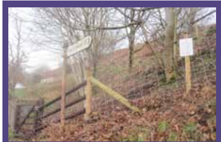
Unlawful fencing on Melinbyrhedryn Common, nine kilometres south-east of Machynlleth in Powys, photographed by one of our members in January. Thanks to the member's efforts and those of Powys County Council, the owner has now removed the fencing, leaving only the wooden posts.
