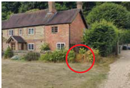
Ranger's Cottage with an unlawful gate on the right (encircled), preventing access to the common. Google streetview.
