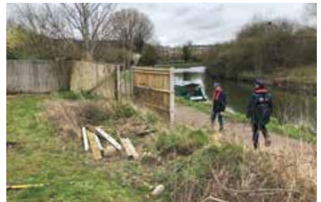
The fence being removed. Photo used with permission of CRT.
