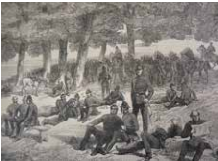
Police on Wanstead Flats, July 1871. Credit: British Newspaper Archive.
