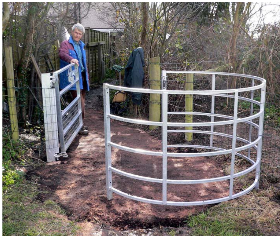
After (viewed from opposite direction). Here the RADAR (Royal Association for Disability and Rehabilitation) lock system is being demonstrated to show how a RADAR equipped gate can be opened past the closure point to allow larger electric wheelchairs to pass.
